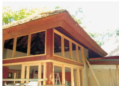
The Progress of job at Fijian Resort Chi Spa
